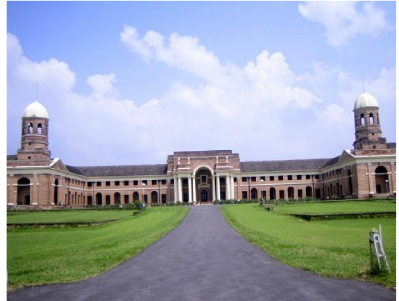
Pic 2. FRI main building
